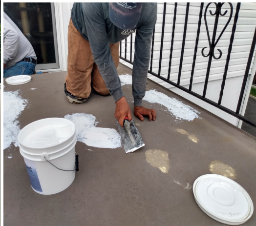
Using Brushable Sealant to smooth out the blemishes
