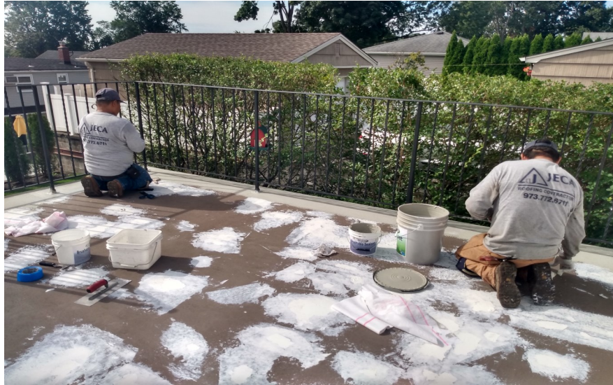
Installing 12" fabric around perimeter and details
