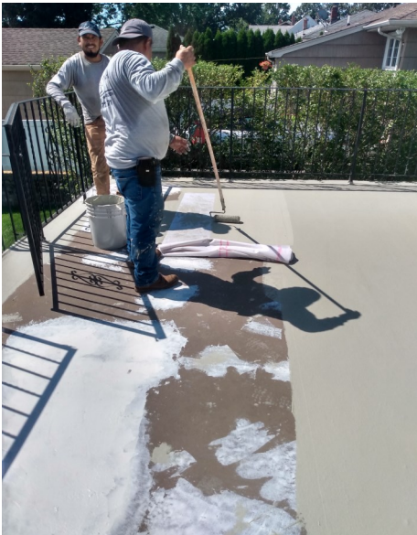
Installing Acrylabs Base System
