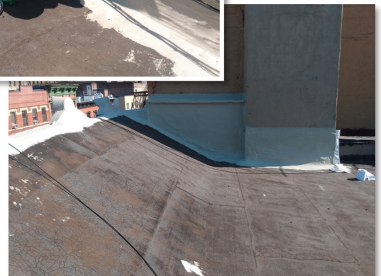
Sealed with Fabric Reinforcement around all bulkheads, parapet walls, and pipes
