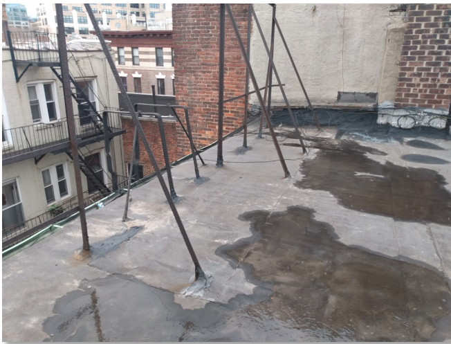
Acrylabs Asphalt Emulsion applied to all low spots
