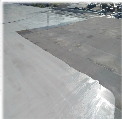
Finish Coat over Base System over Mod Bit
