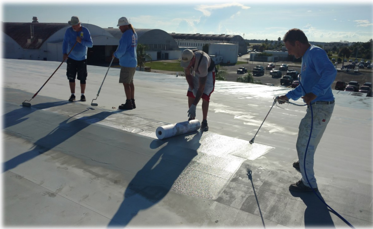
Spray Technique Installing Fabric
