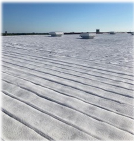
Finish Coat over PUF over Metal
