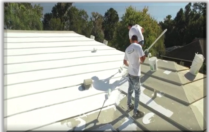
Applying Finish Coat on top of Acrylabs Base System
