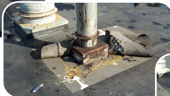
Removing damaged EPDM to expose ISO board
