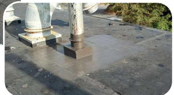
Acrylabs Full System. Using Acrylabs Bronze Finish to match the weathered and faded EPDM.
