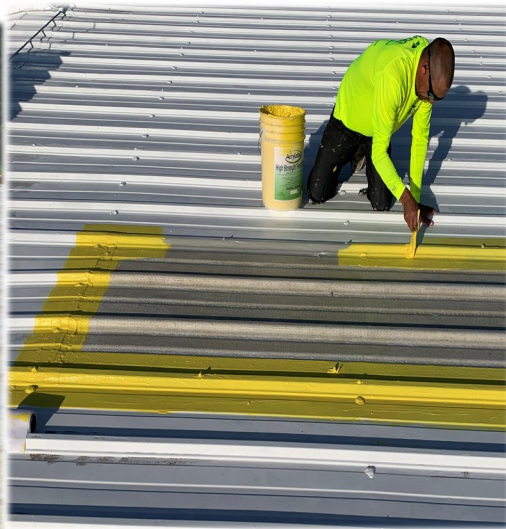
Contractor applying Safety Yellow around perimeter of Sky light making it more visible and safe
