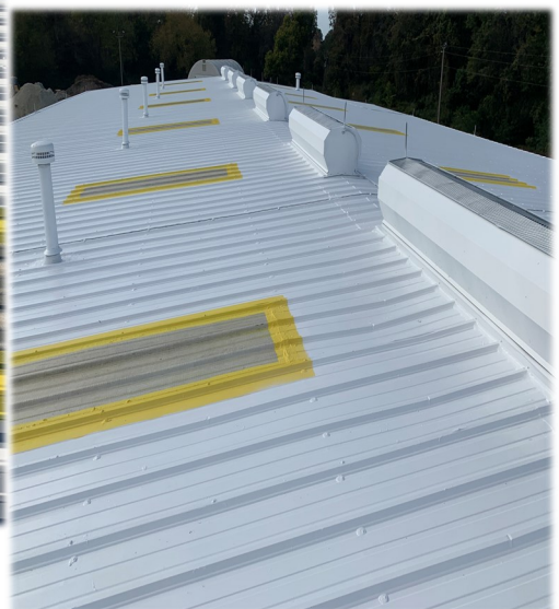
Contractor applying Safety Yellow around perimeter of Sky light making it more visible and safe
