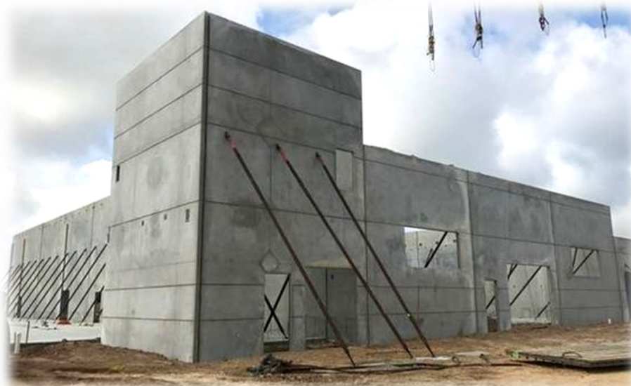
Tilt up concrete structures treated with Acrypel to keep out water and moisture
