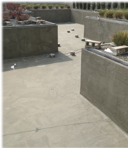
Completed Acrylabs Base System with Acrycrete applied to floor and walls
