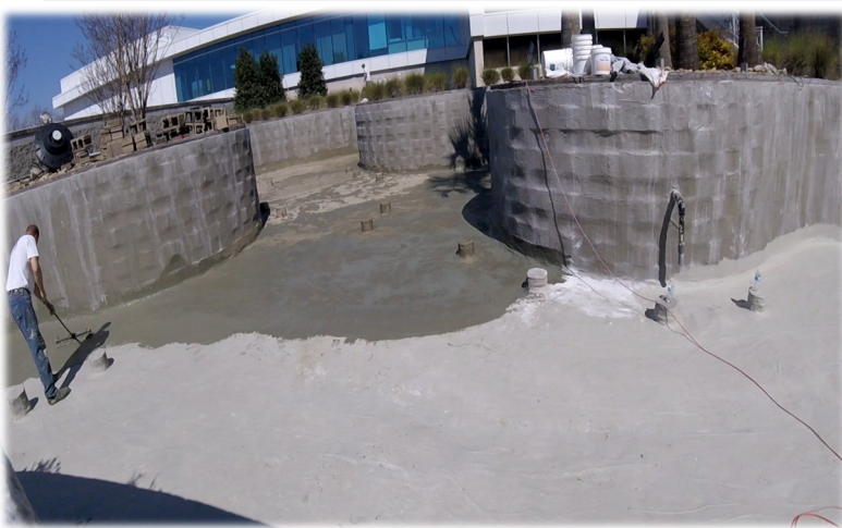
Applying Acrylabs Acrycrete cementitious coating
